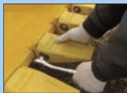
Set bushing, washer and bolt and tighten by a ratchet wrench
